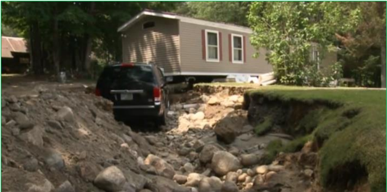
Damage to home on Sculptured Rocks Road, July 2019
